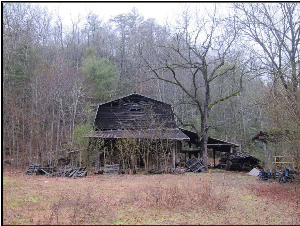
Figure 10. Gambrel roof barn, facing northwest.
