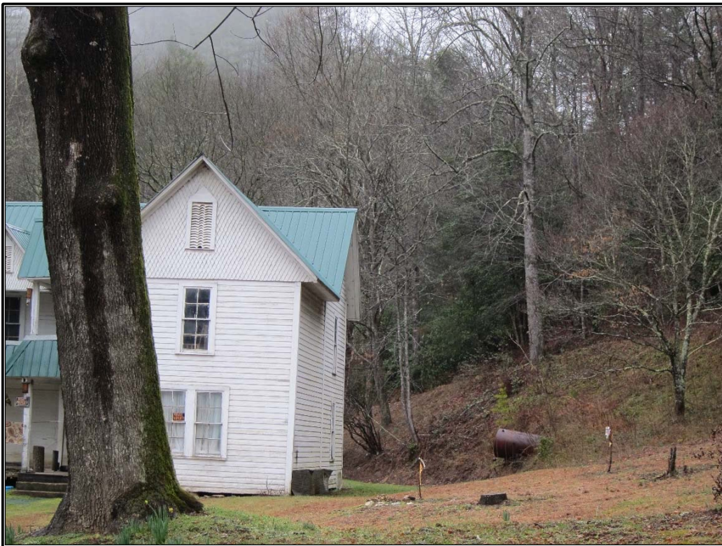
Figure 6. Northeast elevation, facing northwest.
