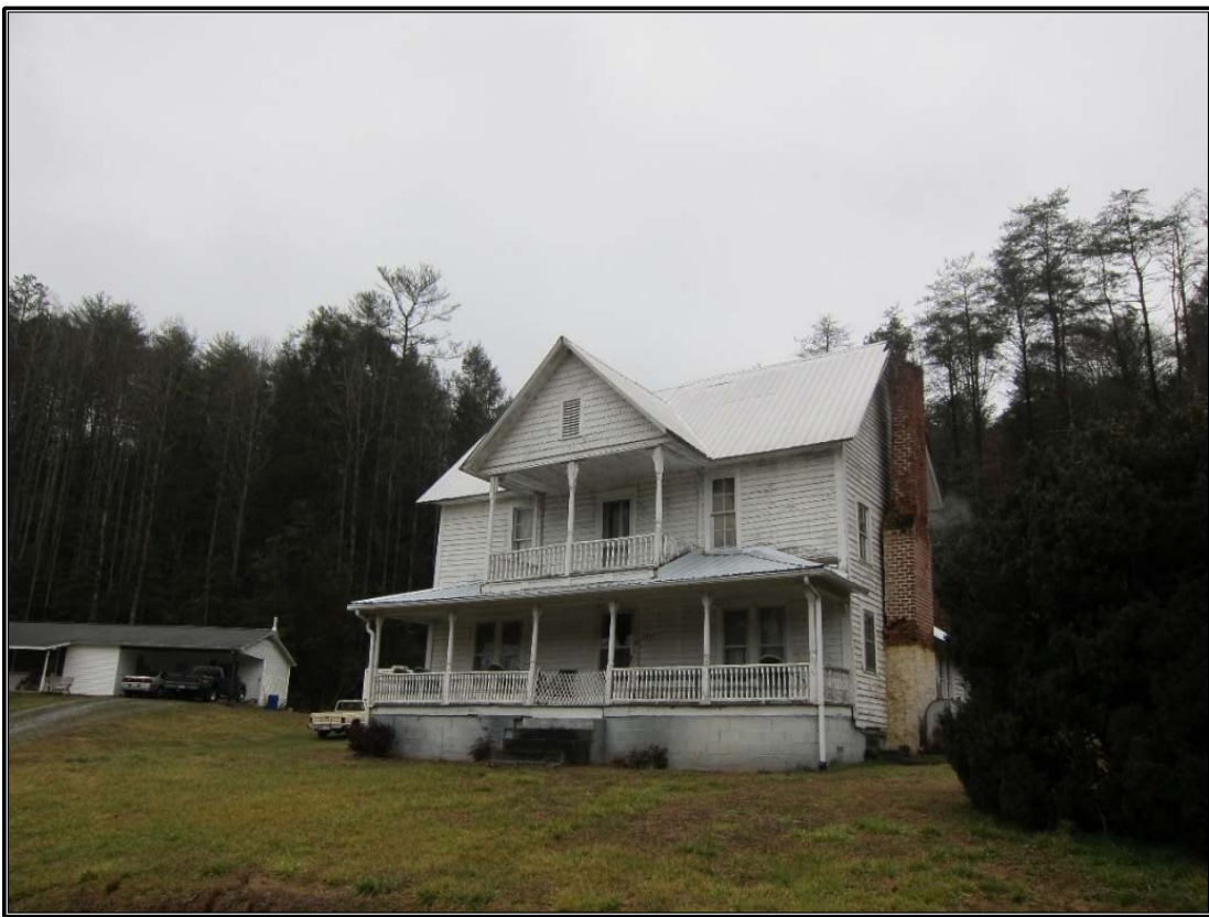
Figure 14. Comparative example located at 2827 Old Johns River Road, facing north-northwest.
