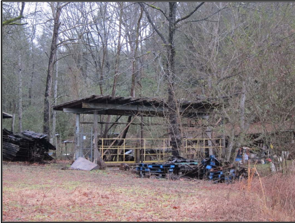
Figure 9. Metal stringer footbridge over Elijah Estes Mill Creek, facing north.
