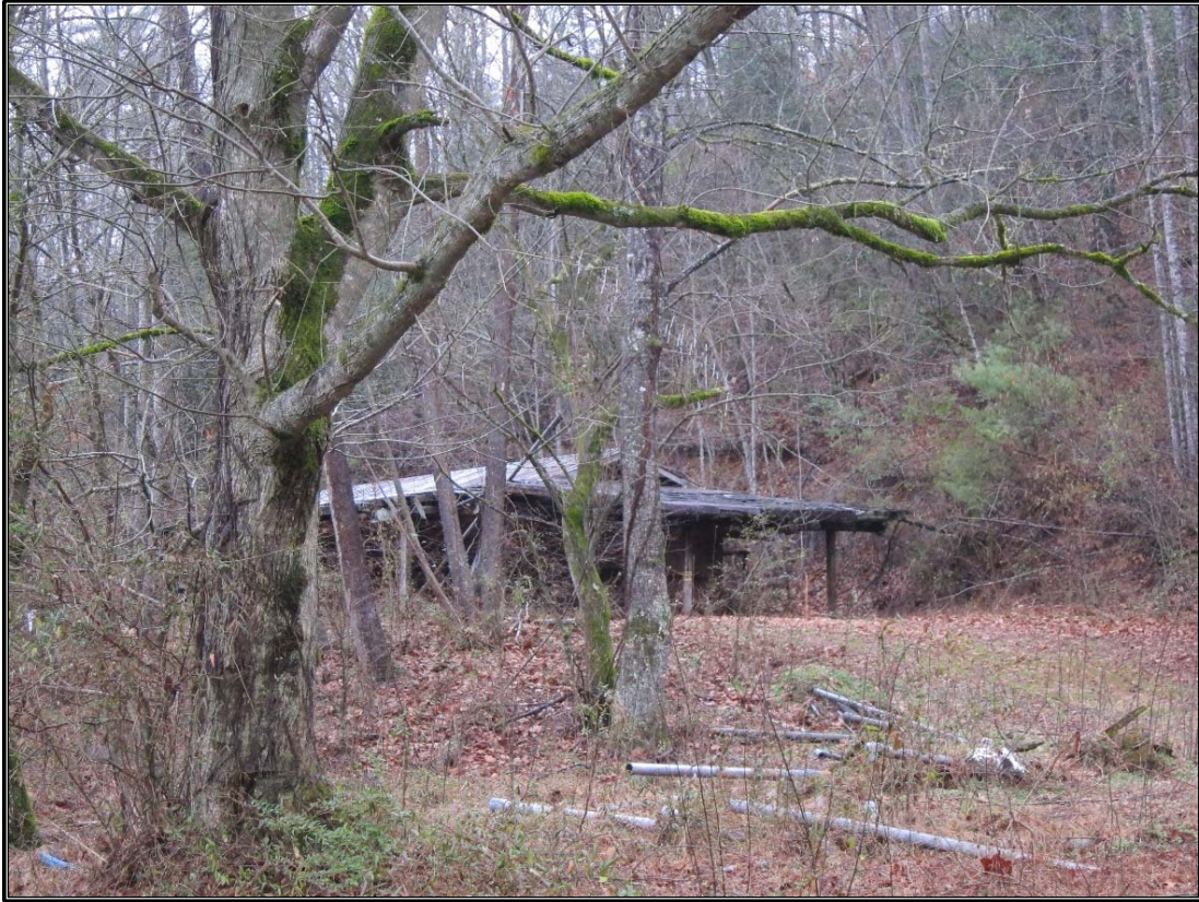
Figure 11. Shed, facing west.
