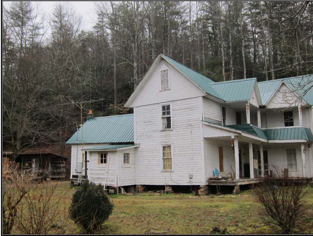
Figure 7. Southwest elevation and additions, facing north.
